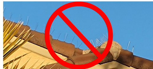
Spikes attached to points along roofline ARE NOT PERMITTED!
